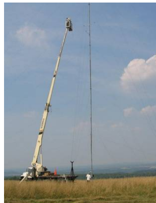
Boom truck used to mount pulley system
